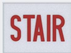
Stair Exit Sign
