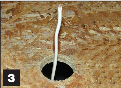
Figure 3 - Pull NM Cable through floor. Figure 3 - Tirer le câble NM à travers le plancher. Figura 3 - Jale el cable NM a través del piso.
