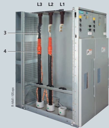
Cable connection compartment with cable termination
