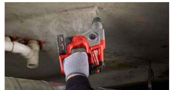
**1/2" SDS Plus Rotary Hammer Kit**
